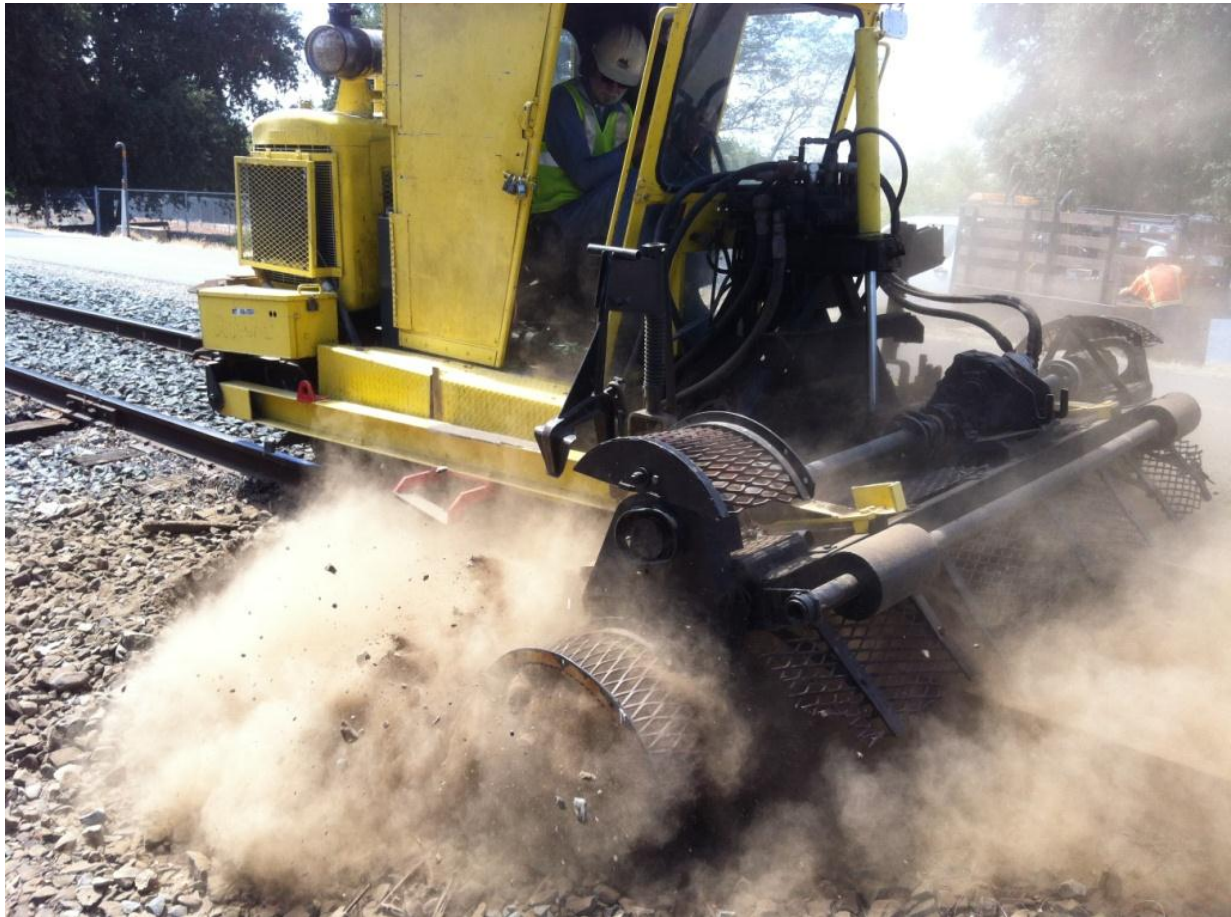
The scarifer scarifying...
