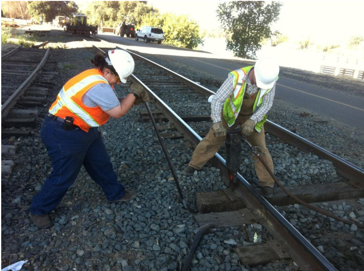
Heather nips the tie while DJ spikes with the pneumatic spiker
